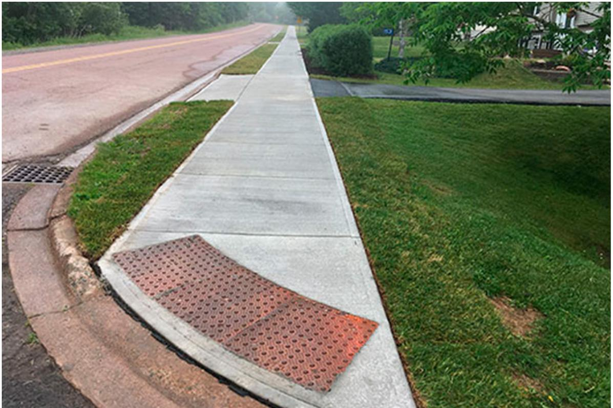
Figure A.4. Sidewalk with tactile warning surface. (Source: Colchester, CA)
